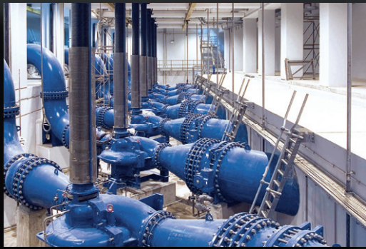
Pumps and compressors
