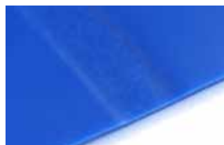
Overlap welding with hot press
